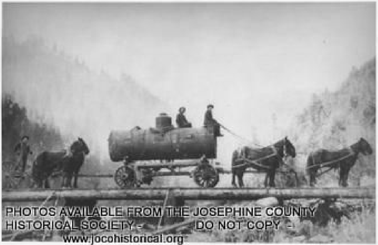
Boiler across footbridge to Almeda Mine
