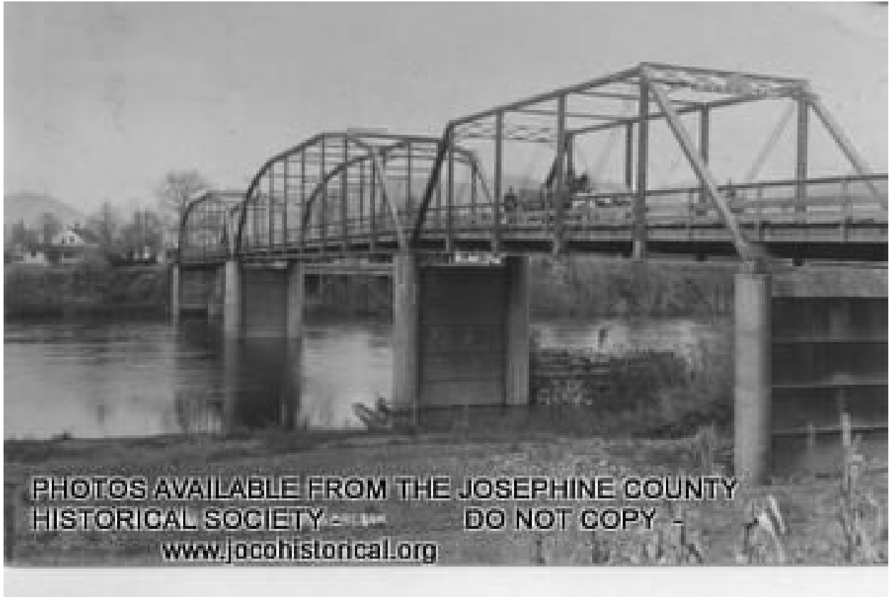
Three Span Bridge at GP new in 1909 photo 1917
