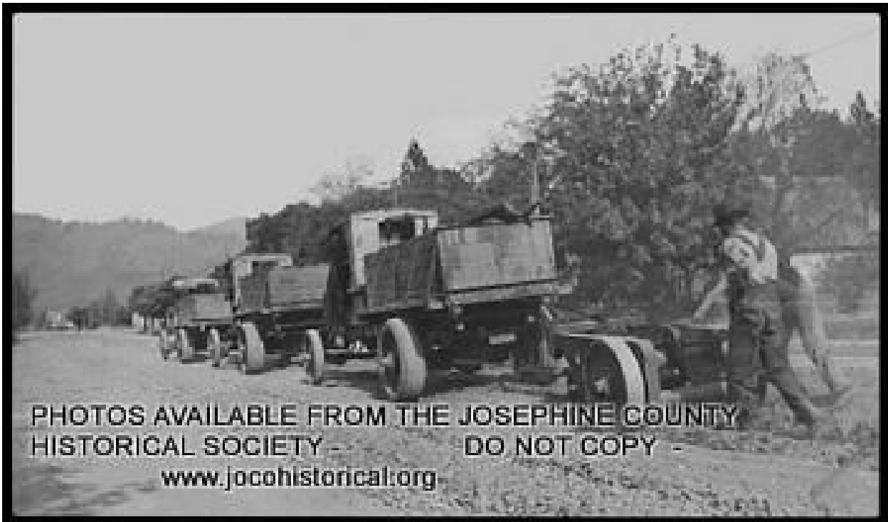
Trucks & scarifier with two yds gravel to stop spinning
