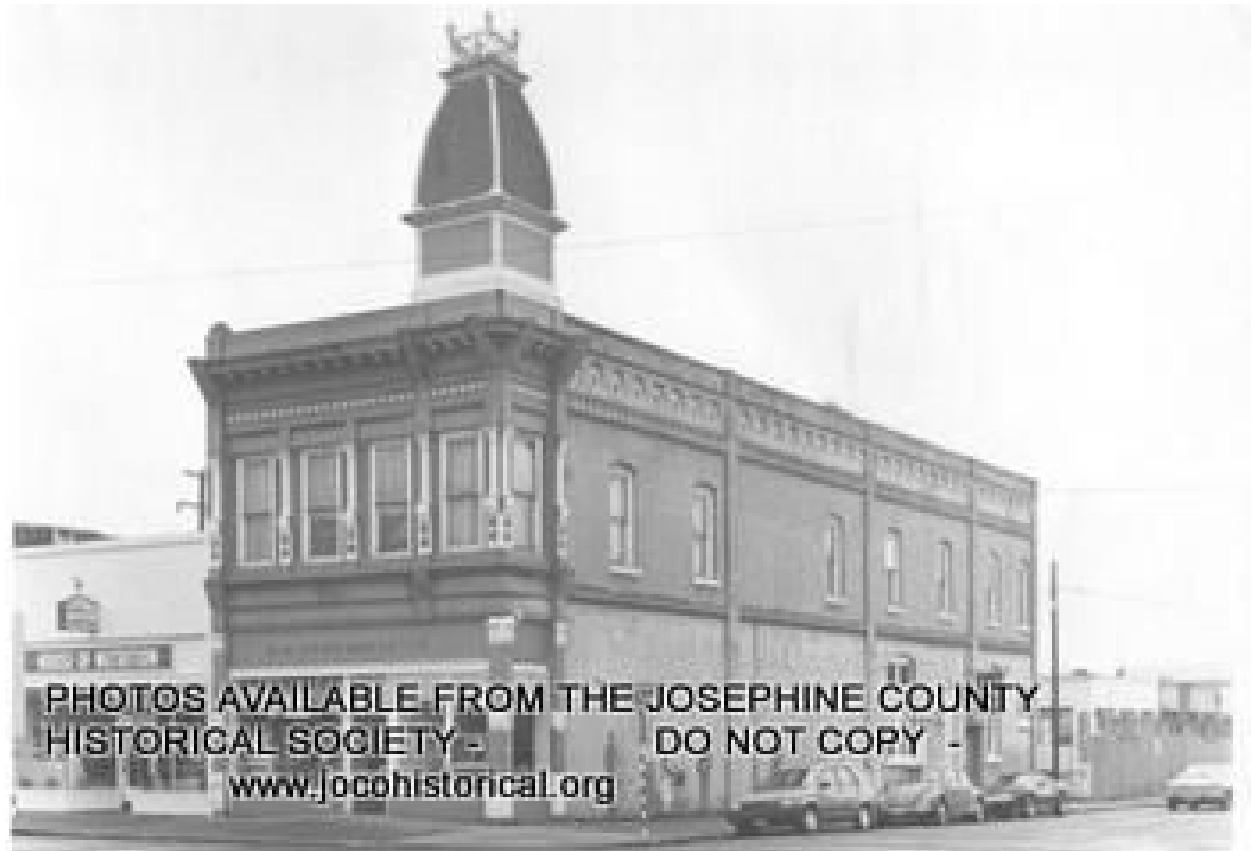
Towers of G.P. 005
