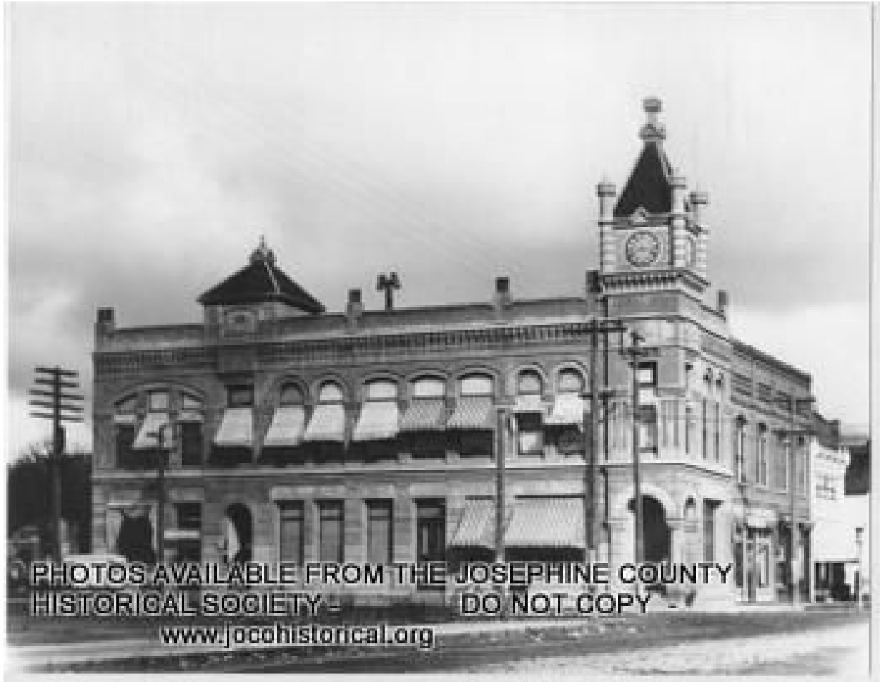
Towers of G.P. 008
