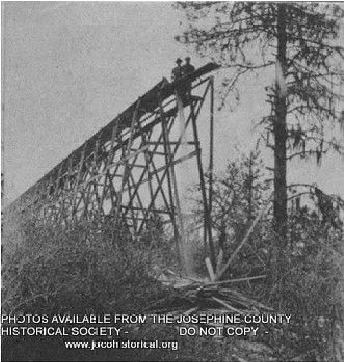
Three Pines lumber flume being repaired
